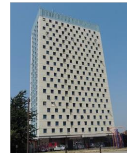
Enfield Walbrook House
