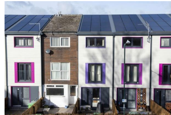
The UK's first Energiesprong project in Nottingham is an example to follow but it also highlights the problem which leasehold tenure can present in retrofit projects, undermining both the technical and architectural ambition here. For multistorey schemes, leaseholders can potentially block entire projects especially where the planned improvements are reliant on external re-cladding (© Mellus Homes).
