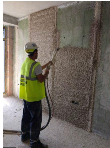
Wet applied insulating plaster
