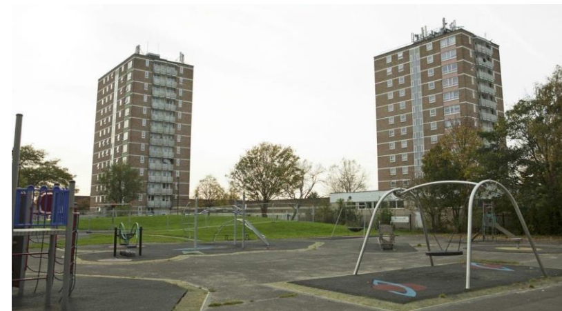
The Channel Island / Exeter Road estate in Enfield has been retrofitted with a communal ground array and individual water heat pumps in each unit.
