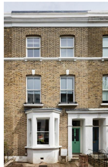
An example of a house fitted with various enhanced glazing. New double-glazed sashes on the second floor, secondary glazing to the first and new double glazing into old frames on the ground.
