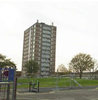
Channel Islands Estate, Enfield
