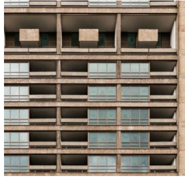
Balfron Tower, Tower Hamlets
